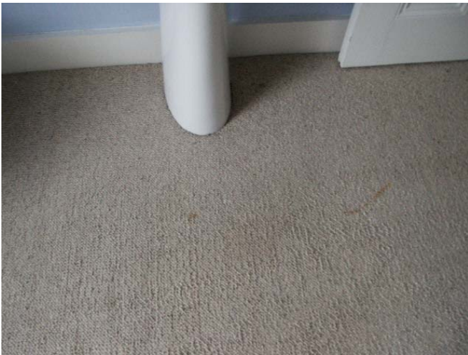
Bathroom – stains to carpet
